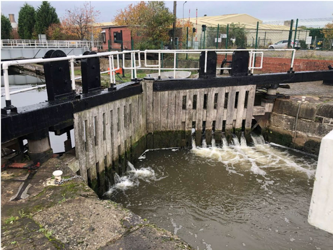
Figure 3 - Downstream face of the top lock gates to be modified at Keadby Lock (image Arcadis 2022)
